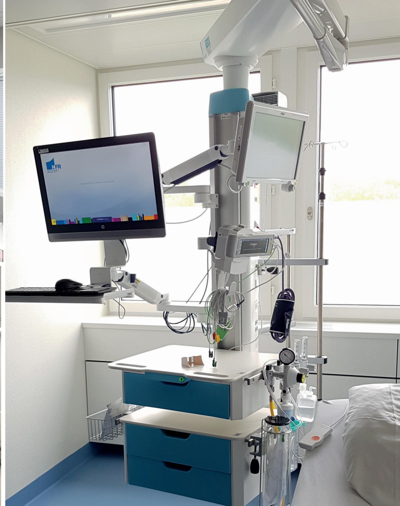
Service des Urgences, Hôpital de Fribourg, Suisse Emergency Department, Friborg Hospital, Switzerland
